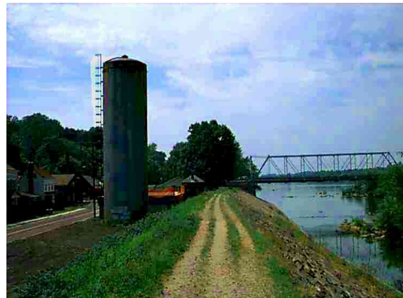
View of the Calhoun Street Bridge from the River Dike
